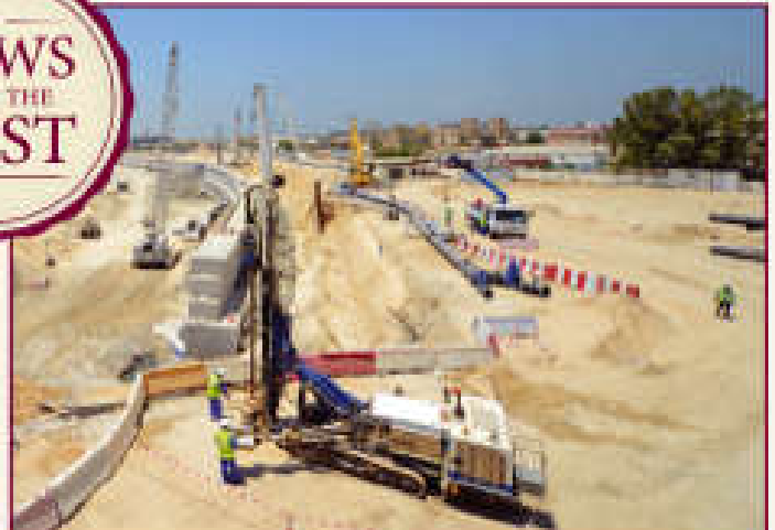
Lovejeet Singh, Subeer Khan (Technician) and Muhammed Riyas (Banksman) installing the main 630 mm HDPE pipeline.
