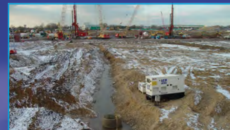
Heathrow Terminal 5 open trench and sump pumping in Terrace Gravels
