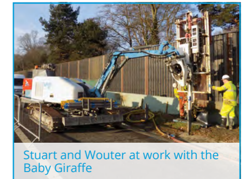
The Baby Giraffe & SM10 drilling rigs at work
